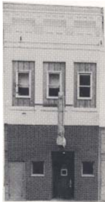
Existing Modified Storefront
